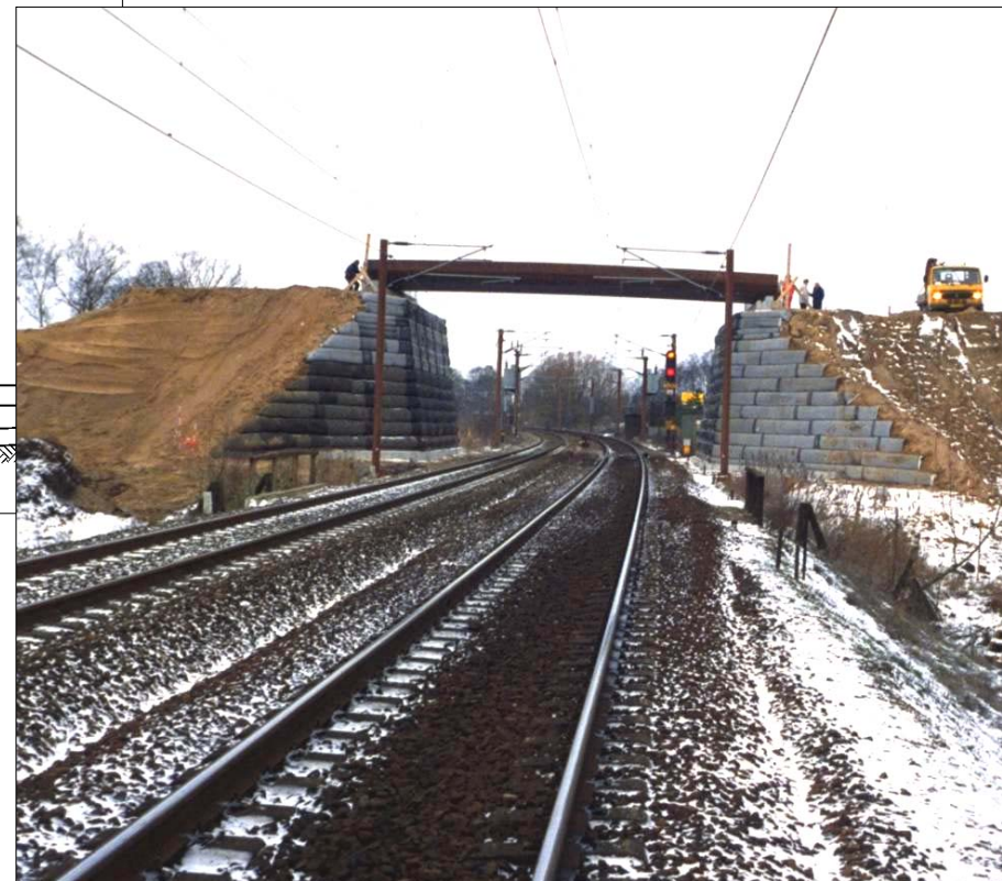
Bridge abutments at Ullerslev, Denmark, 1991 May be the first geogrid-reinforced bridge abutment in Europe
