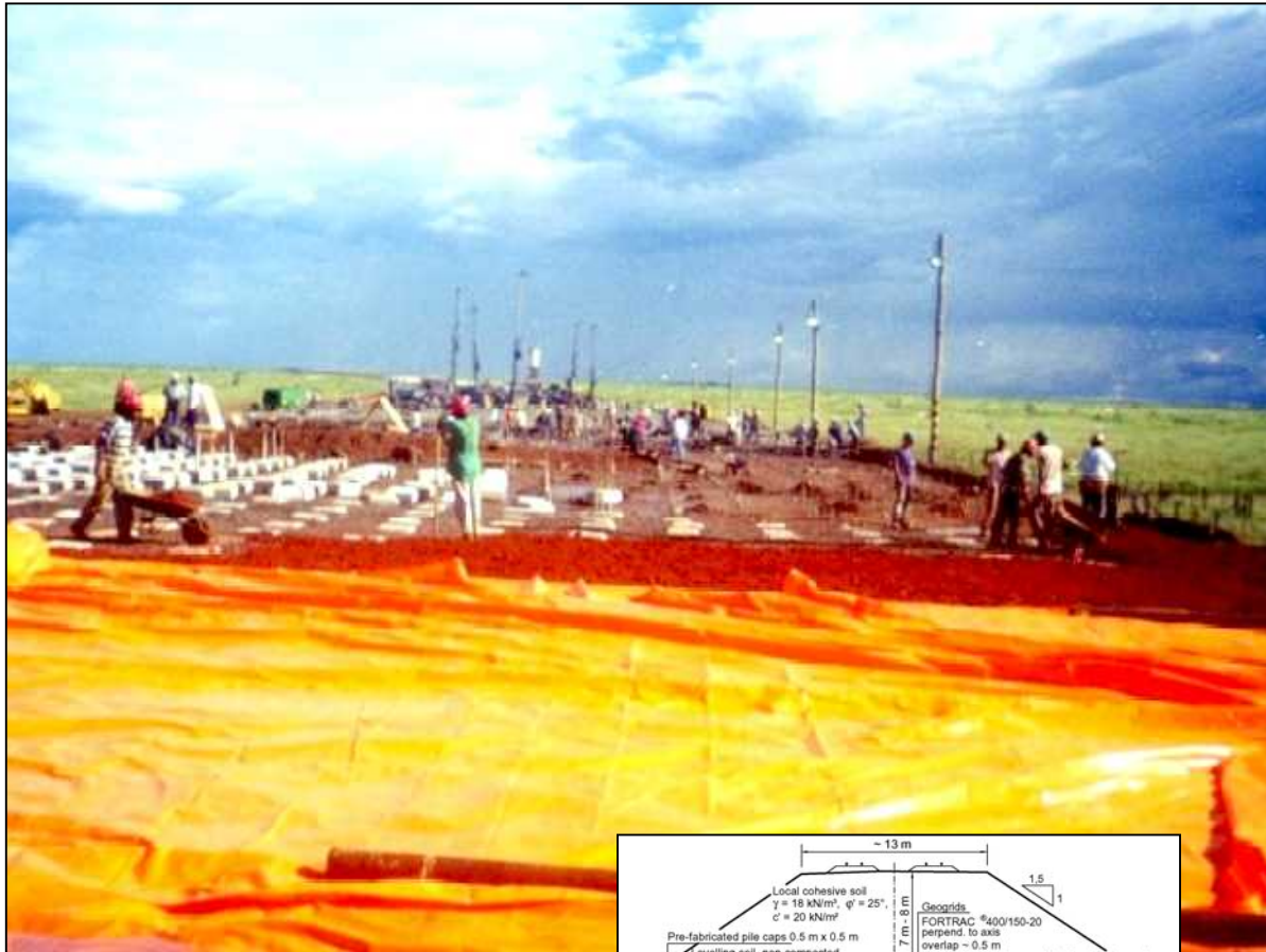
Ferronorte, River Laje at Chapadao, Brasil, 1998, semi-biaxial geogrids FORTRAC 400/150
